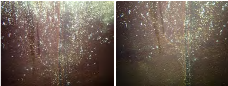
Upper West Wall Section- Photo of weld deficiencies
