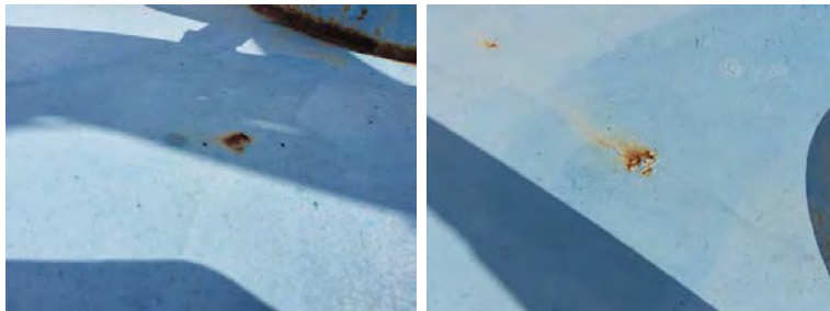
North Quadrant- Photo of weld deficiencies
