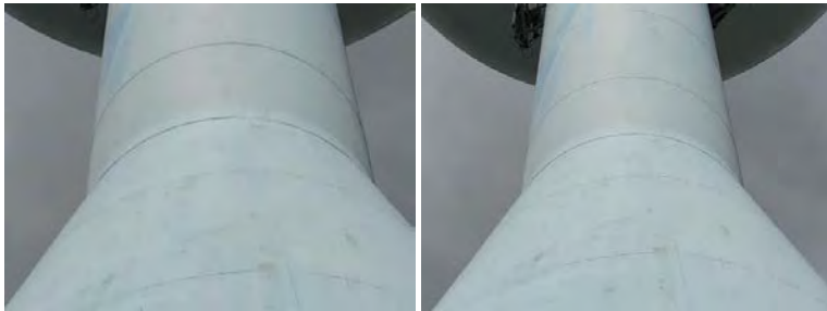
Upper South Wall Section- Photo of welds
