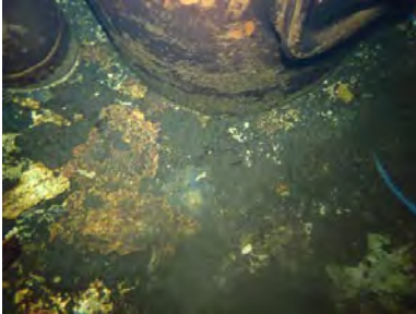
Overall Photo of Interior South Floor Quadrant
