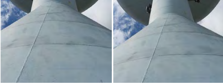
Middle East Wall Section- Photo of welds
