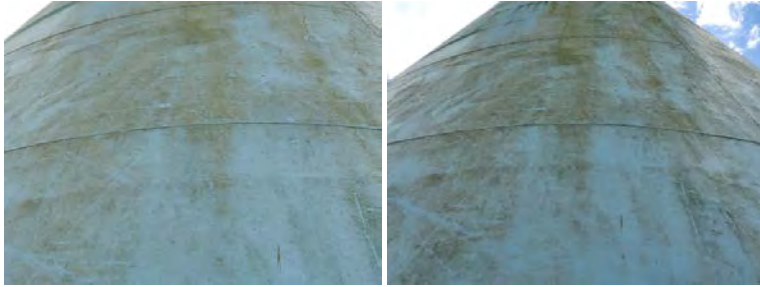
Middle North Wall Section- Photo of welds
