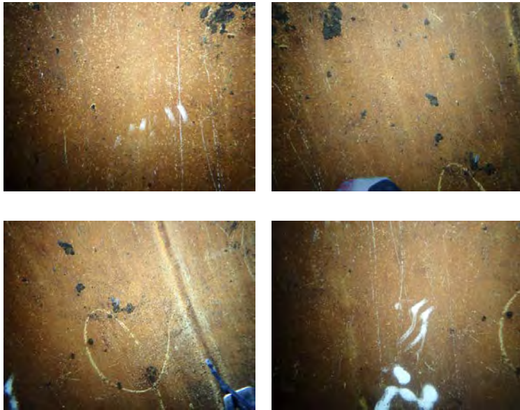
North Floor Aesthetics Photos
