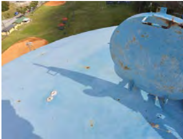
Photo of exposed steel
