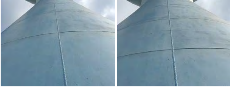
Middle West Wall Section- Photo of welds
