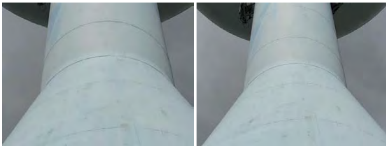
Upper South Wall Section- Photo of welds
