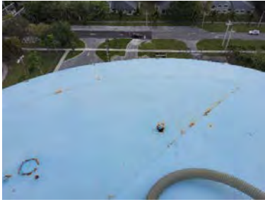
Photo of exposed steel
