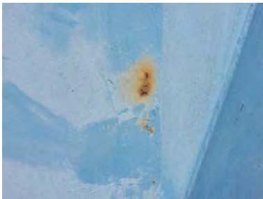
Photo of exposed steel
