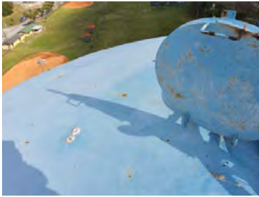
Photo of exposed steel
