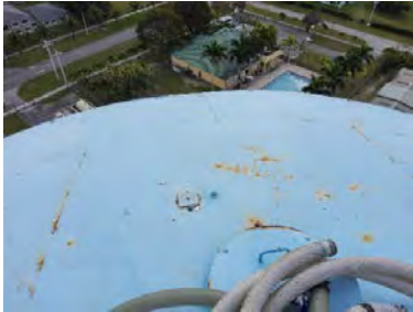
Photo of exposed steel
