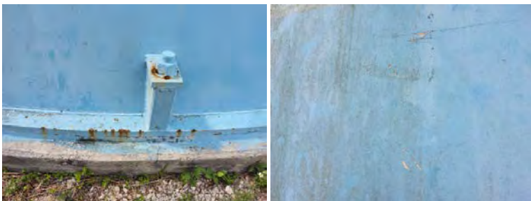
Photo of exposed steel
