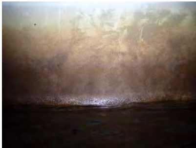
East Wall Aesthetics Photos
