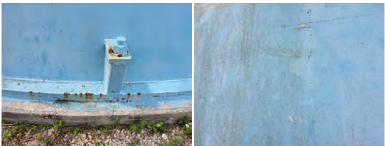
Photo of exposed steel
