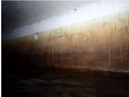
Overall Photos of Interior East Wall Quadrant
