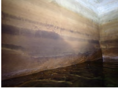
Overall Photo of Interior South Wall Quadrant
