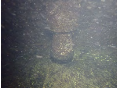
Column #4 Photo of corrosion
