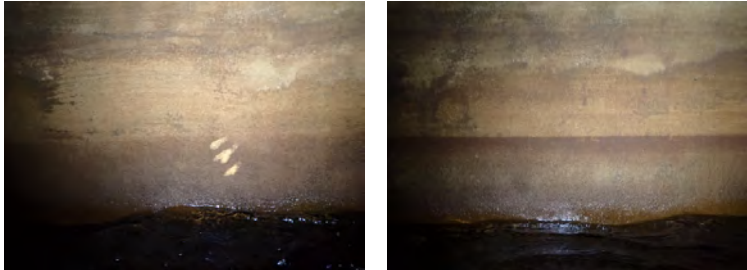
East Wall Aesthetics Photos
