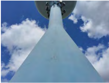
Photo of exposed steel
