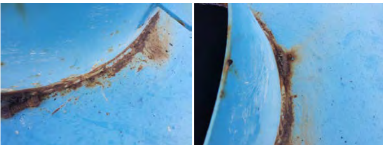
North Quadrant- Photo of weld deficiencies
