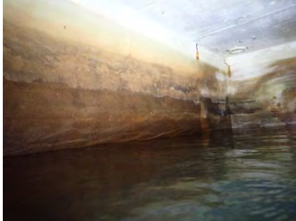
Overall Photos of Interior West Wall Quadrants
