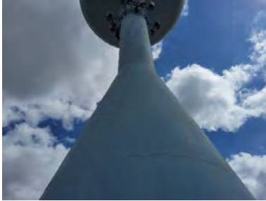
Photo of exposed steel
