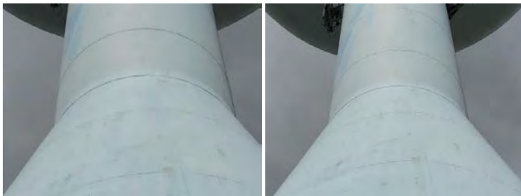
Upper South Wall Section- Photo of welds
