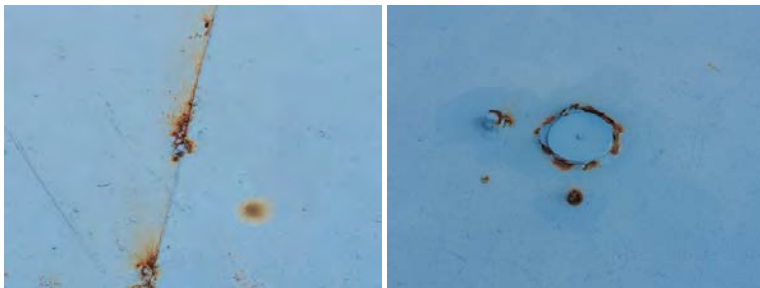
East Quadrant- Photo of welds
