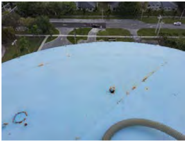
Photo of exposed steel
