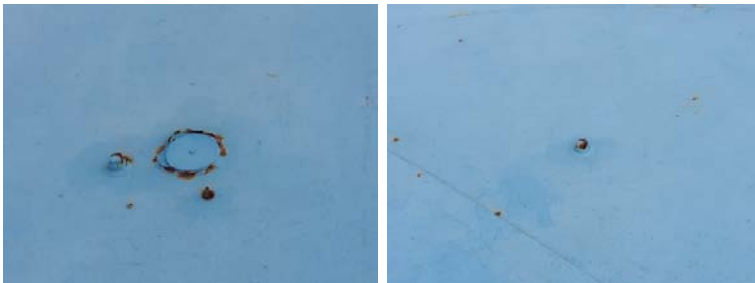
Photo of exposed steel
