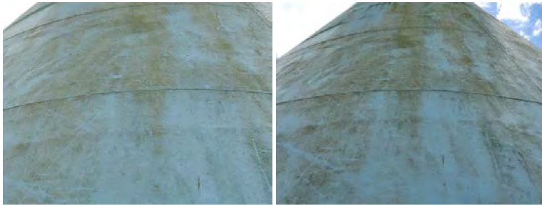
Middle North Wall Section- Photo of welds
