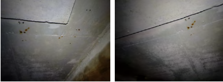
South Overhead Aesthetics Photos
