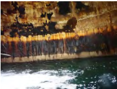
Interior Upper North Wall Section- Photo of corrosion
