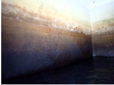
Overall Photo of Interior North Wall Quadrant
