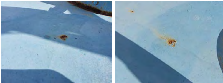
North Quadrant- Photo of weld deficiencies
