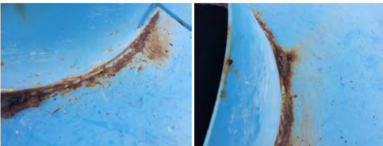
North Quadrant- Photo of weld deficiencies
