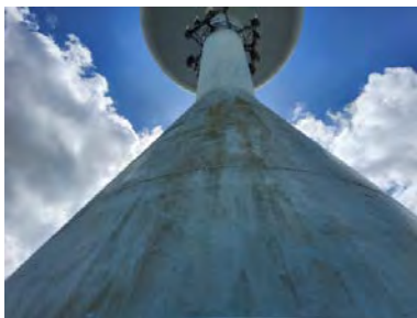
Overall photo of this quadrant
