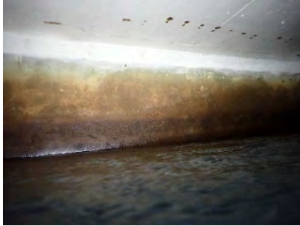
Overall Photo of Interior South Wall Quadrant
