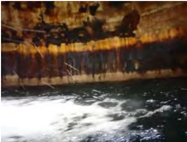
Interior Upper North Wall Section- Photo of corrosion
