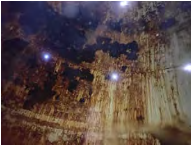
Overall Photo of this quadrant
