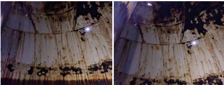
Interior Upper South Wall Section- Photo of corrosion
