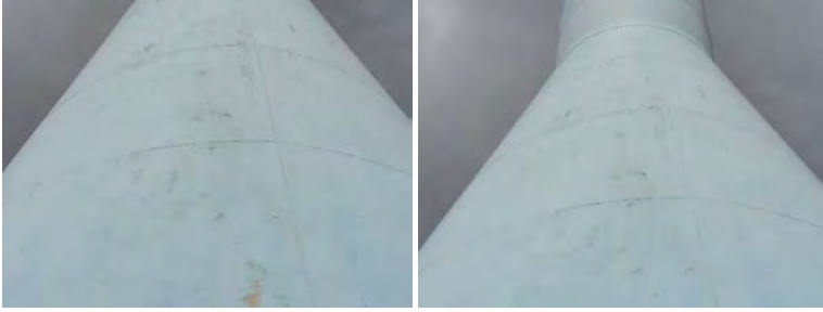
Middle South Wall Section- Photo of welds
