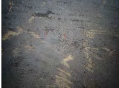
Before Sediment Removal
